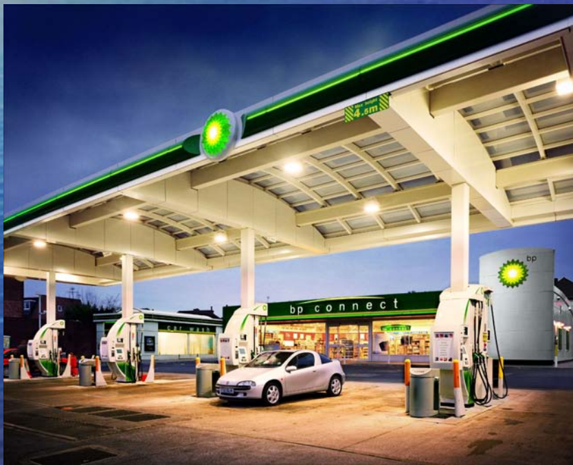
20 KW Solar Roof on Gas Station Canopy
